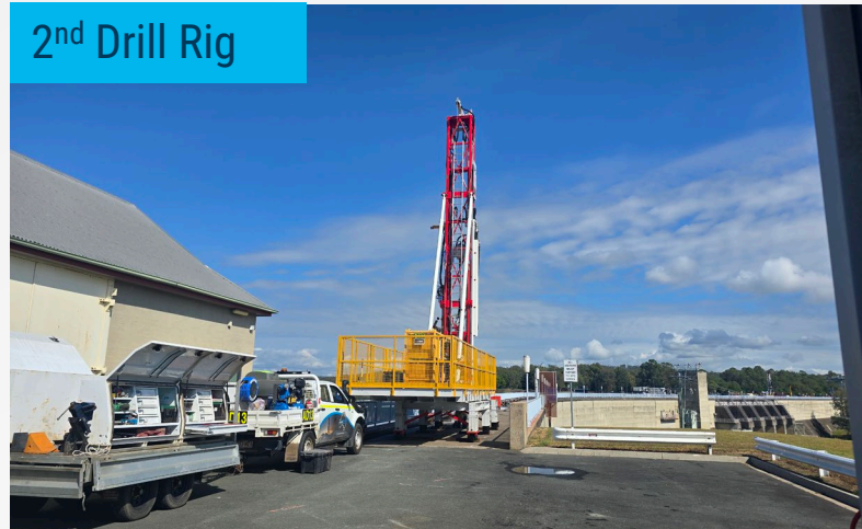
Anchor Grouting
