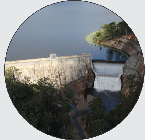
Lake Manchester Dam
