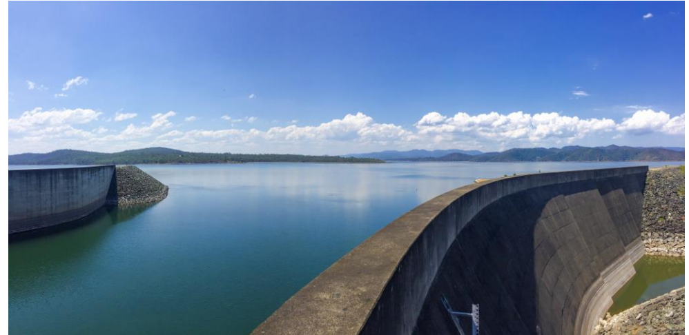
Figure 4: Somerset Dam downstream of dam wall
