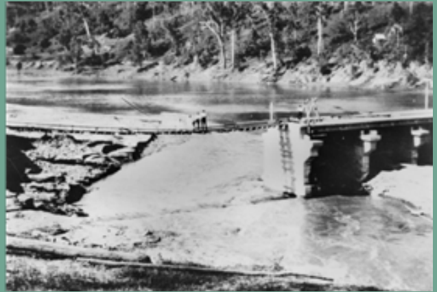
Figure 3: Mt Crosby Weir Bridge damage after 1927 floods. (check source of the photo from Marlee)
