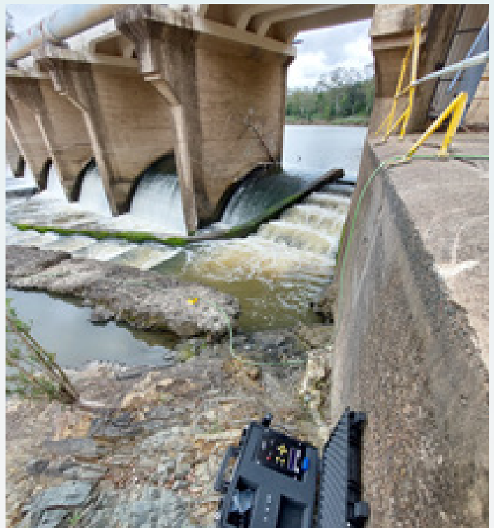
Figure 2: Vibration monitoring in progress on weir bridge.
