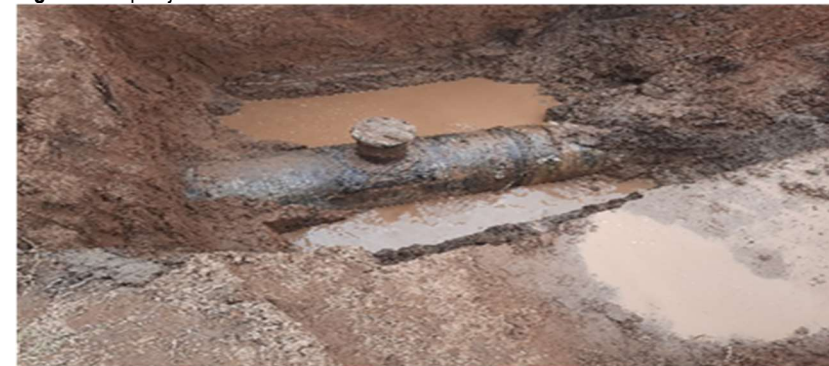
Figure 6: Repair joint.
