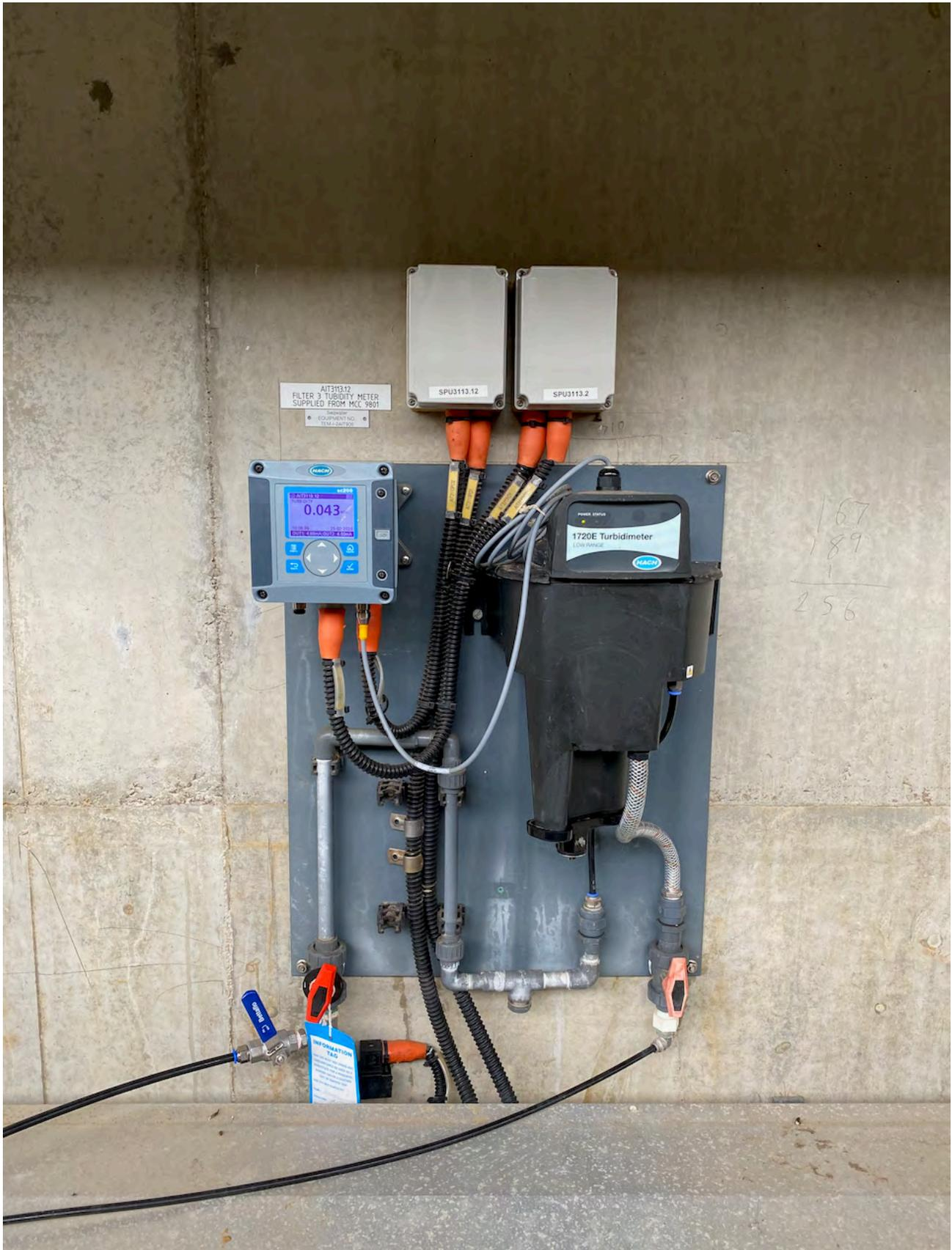
Figure 6-1. Photo of Ewen Maddock WTP turbidity analyser - well labelled and maintained.
