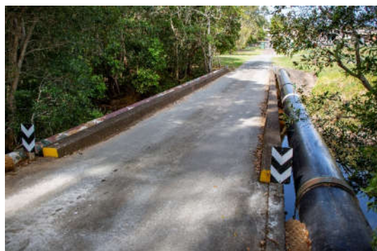
Image: The existing Noosa Water Treatment Plant access bridge
