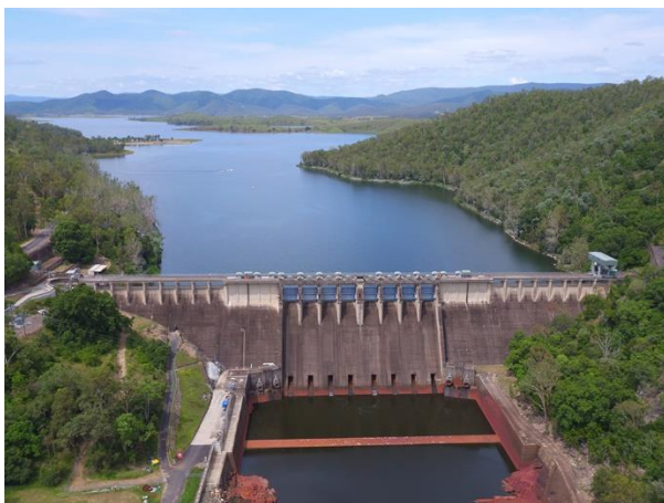
Aerial view of Somerset Dam
