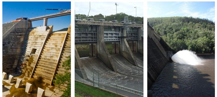
If it rains heavily, or if the river floods, water can escape over a spillway and into the river downstream. This is an engineering design to help remove the water pressure on the dam wall. A spillway is usually built at the side of the dam wall.
