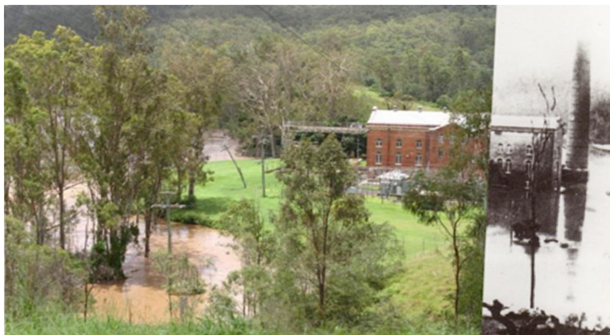
Flooding at the East Bank Pump Station now and then
