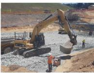
The new pipeline is needed to carry water through the new weighted berm. Maintenance workers will use the access shaft to reach the underground
