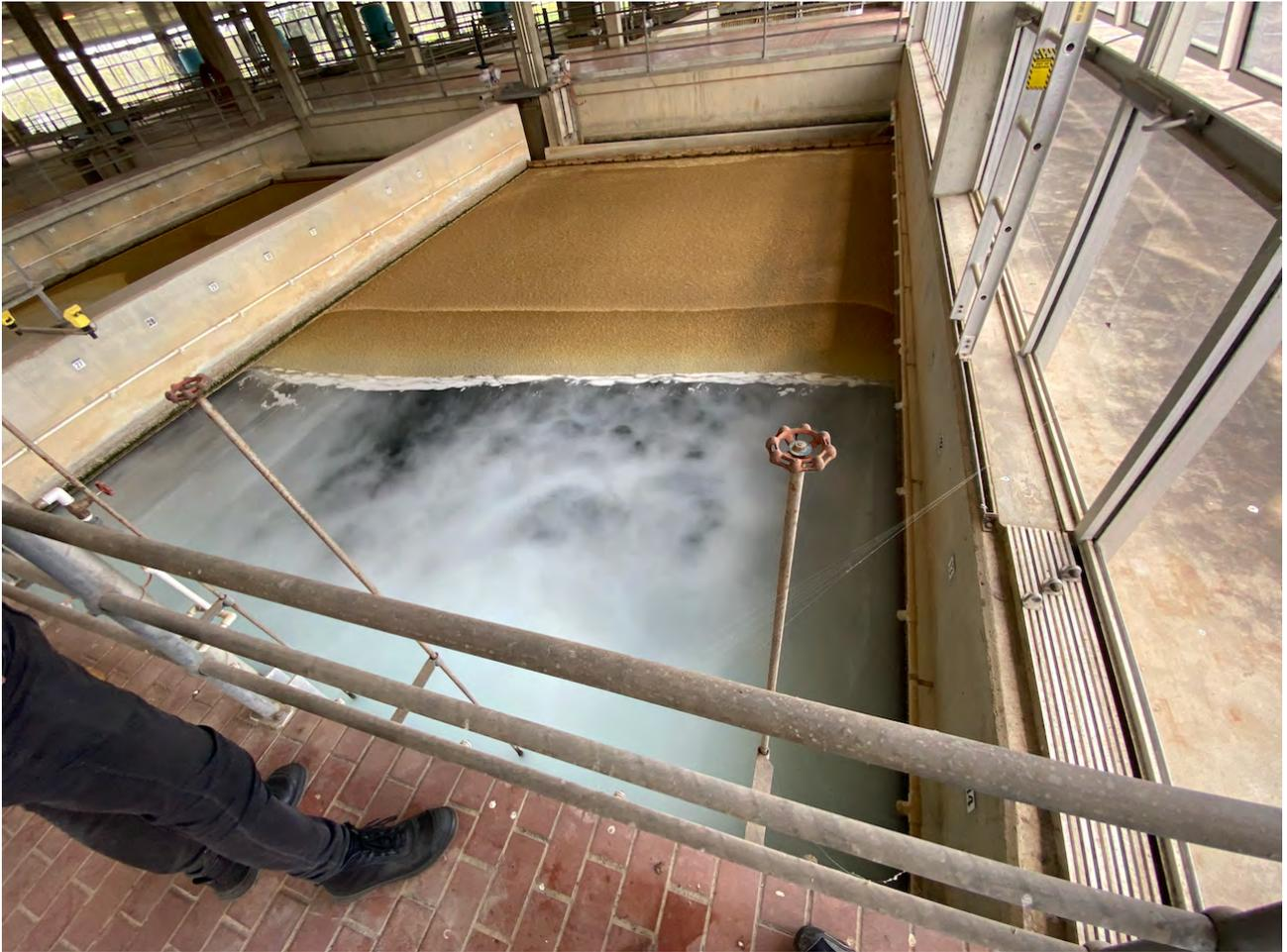
**Figure 6-8. Photo of Mt Crosby Westbank WTP filters – showing excellent inspectability and conditions. The plant was offline during the inspection.**
