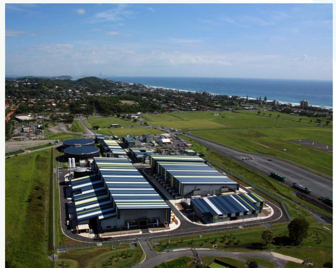
The Gold Coast Desalination Plant uses reverse osmosis to turn seawater into drinking water - a climate-resilient supply of water during drought.
