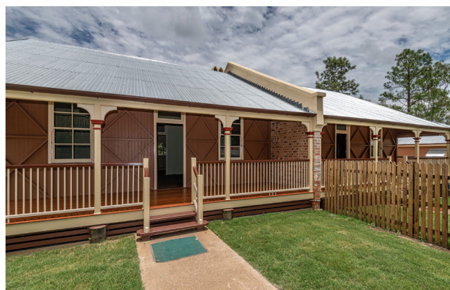
Mount Crosby Duplex Cottages 103 and 104 following refurbishment works
