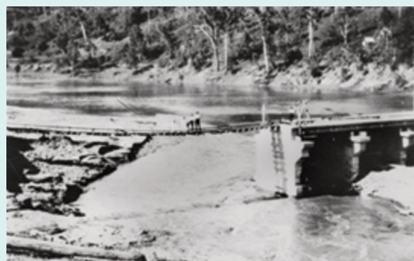
Mount Crosby Weir Bridge damage after flooding
