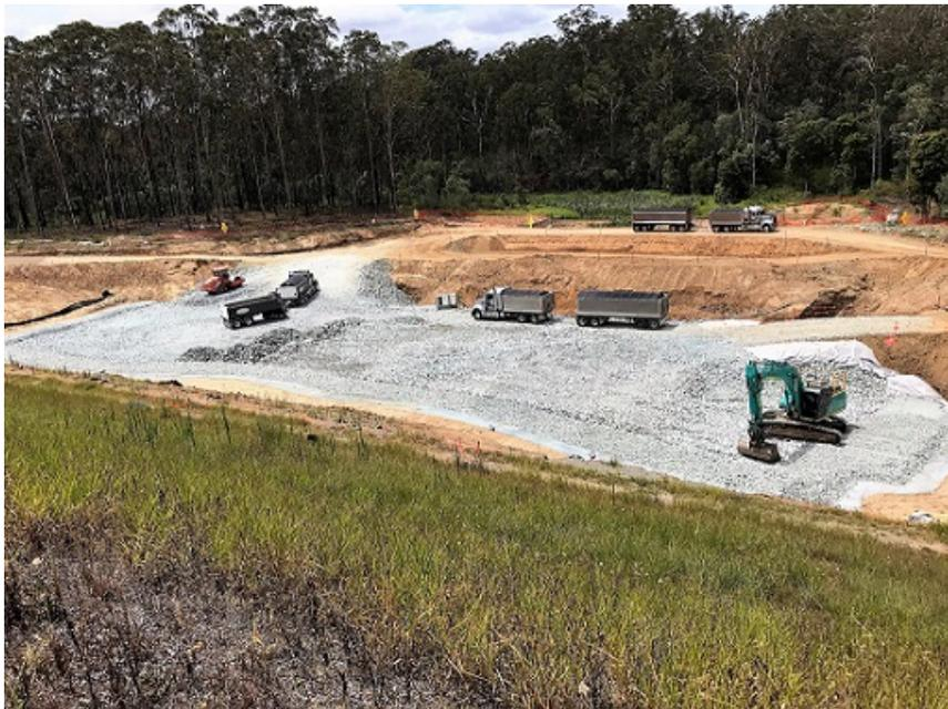
**Image:** Trucks delivering gravel to the main embankment
