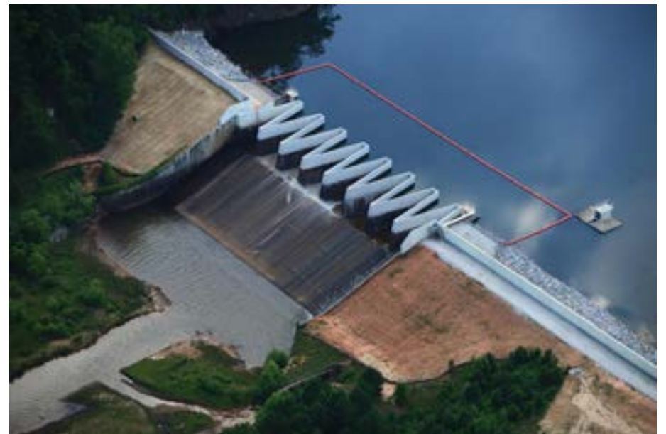
Example concept design of a labyrinth spillway.
