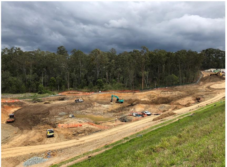
**Image:** Main embankment safety upgrade work
