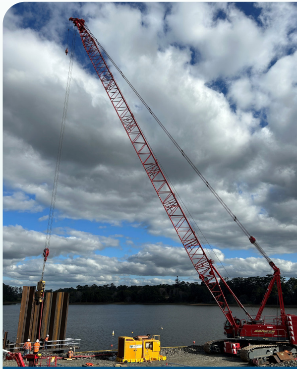
Land piles on the left abutment.
