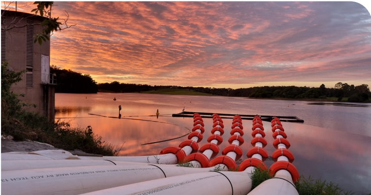
Large siphon system for lake lowering.
