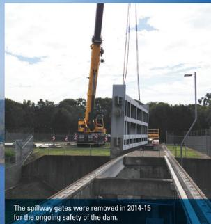
The spillway gates were removed in 2014-15 for the ongoing safety of the dam.
