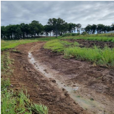
Figure 6: Berm cleaning Pie Creek Scheme
