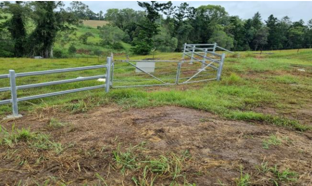
Figure 5: Ongoing fencing upgrade Pie Creek Scheme.
