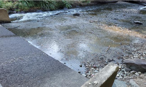
Figure 4: Borumba Weir Measuring flume after repairs.
