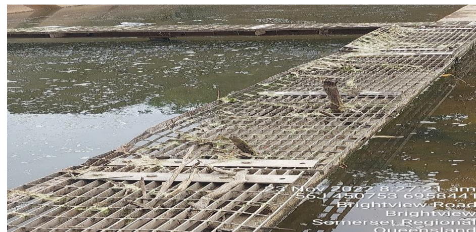
Figure 4: Flood damage to Brightview Weir walkway and hydraulic lines replaced.
