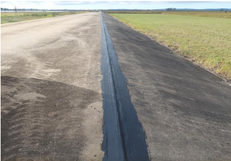
Figure 6: Clarendon Dam spillways repairs
