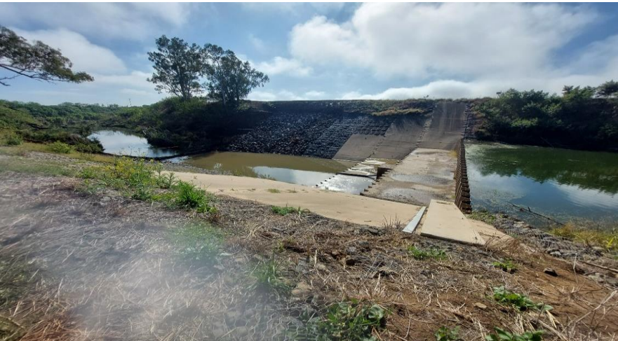
Figure 8: Clarendon Weir flood damage repairs.
