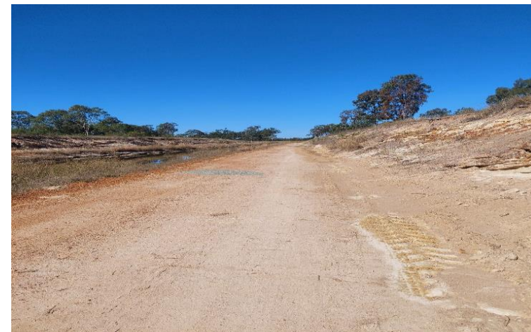
Figure 5: Clarendon channel berm drains cleaned.
