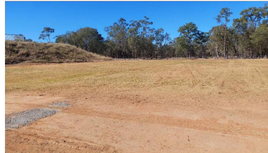
Figure 4: Clarendon channel exposed siphons completed repairs
