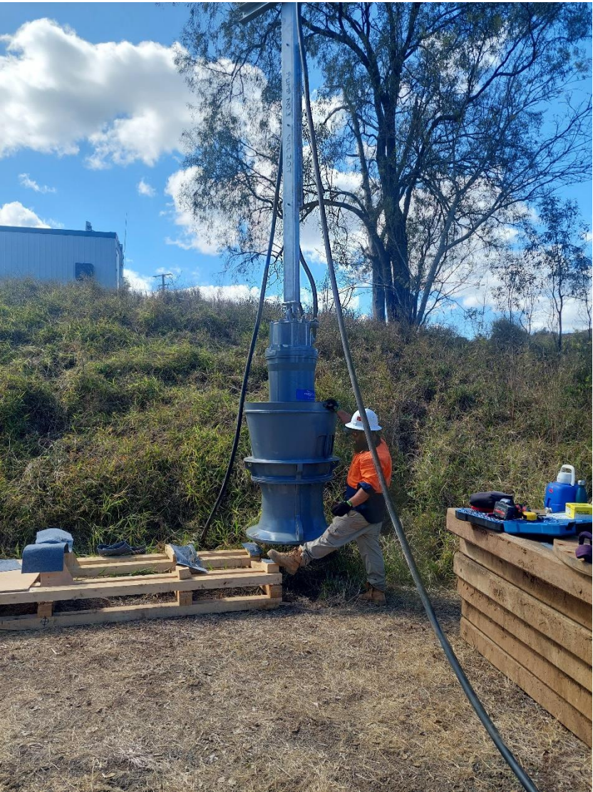
Figure 9: Redbank pump station pump 3 replacement.
