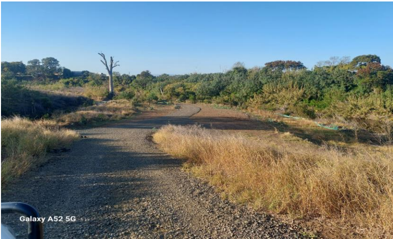
Figure 7: Jordon’s weir access road repairs
