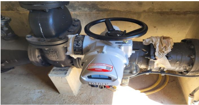
Figure 3: New rotork valve installed Cedar Pocket Dam
