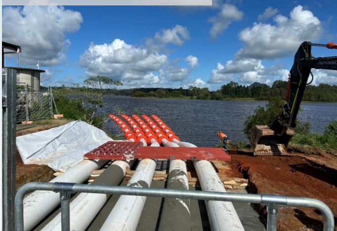
Siphon system installed
