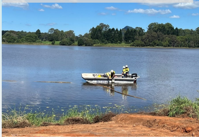
Mitchell Marine installing the site curtain
