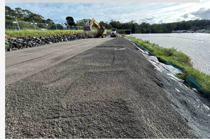
Hardstand 3 ready for crane installation
