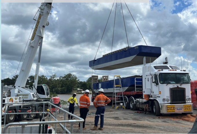
Pontoon for siphon installation
