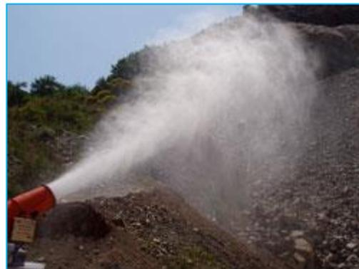
**Spraying a fine mist of water over exposed soil is a common method used to suppress dust.**
