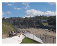
The concrete slab will form the foundation of the extended concrete conduit through the dam wall. This provides a good indication of how much wider the dam embankment will be after construction
