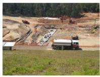
Loose alluvial soils have been excavated, and work has started to widen and strengthen the embankment.
