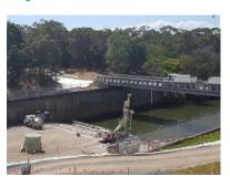
Post-tensioned steel anchors are being installed at the crest of the spillway.
