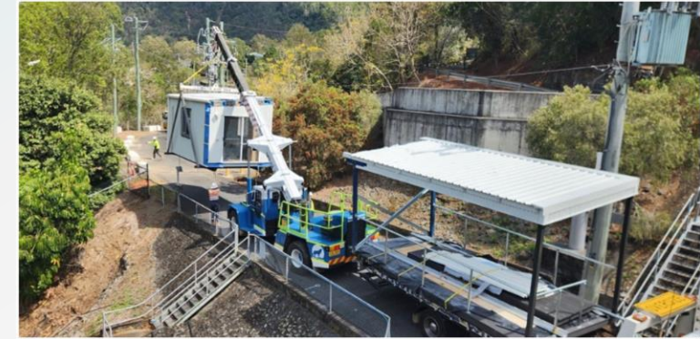
Temporary Operations Facilities
