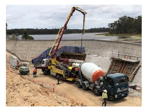
Image: Spillway concrete work
